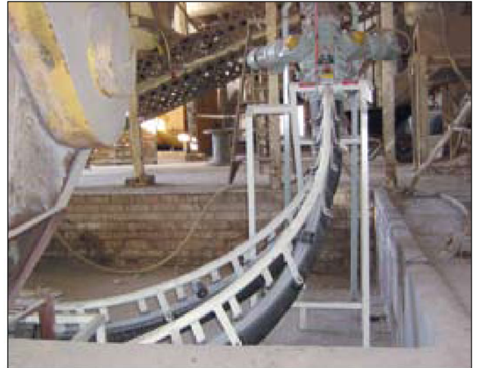
ICS negotiating a 90° compound curve and 1 metre radius.
